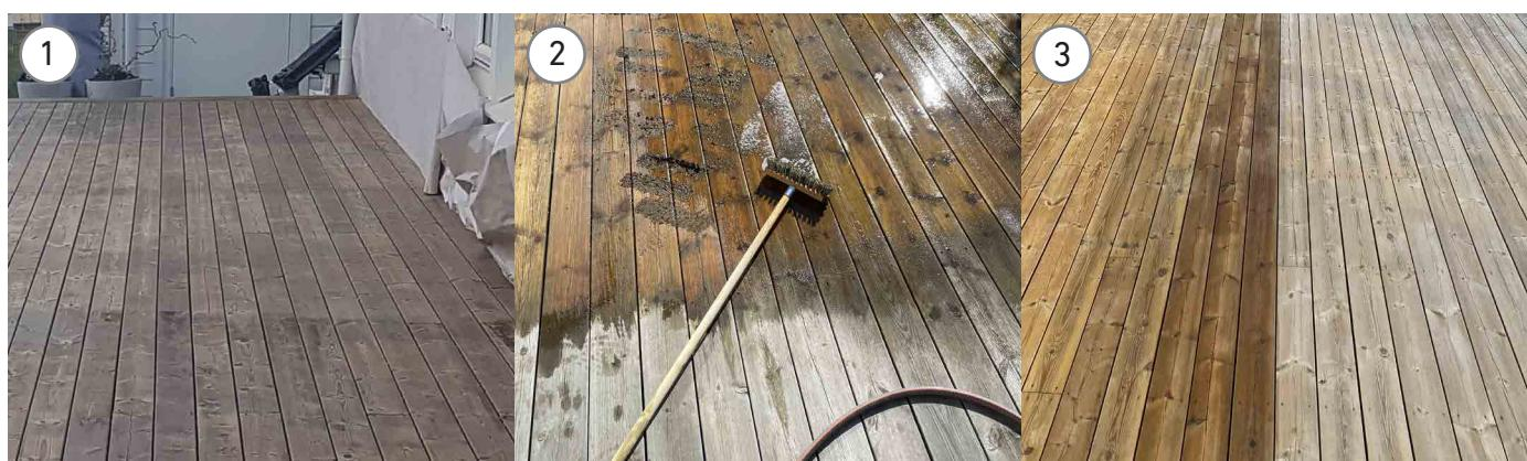
**1 WEEK AFTER.** The colour of the surface may change markedly and also develop some water spots that will gradually disappear with the rain and sunshine. These can be reduced by wet-brushing using water.
