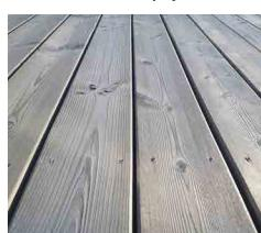
**3–6 MONTHS AFTER.** If the surface has been exposed to both sunlight and rain, a smooth, silver-grey surface will have formed. Maintenance is very simple. Treat the surface with Wood Protection diluted with water at a ratio of 1:1. The treatment further strengthens the wood.
